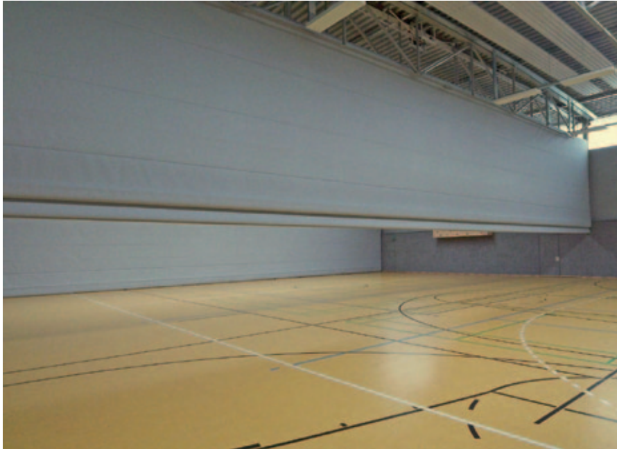
Triple gym with two partitioning curtains extending from wall to wall
