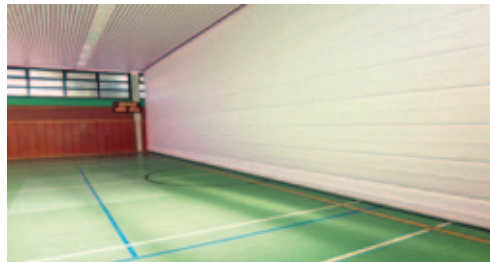
Partitioning curtain for suspended ceiling
