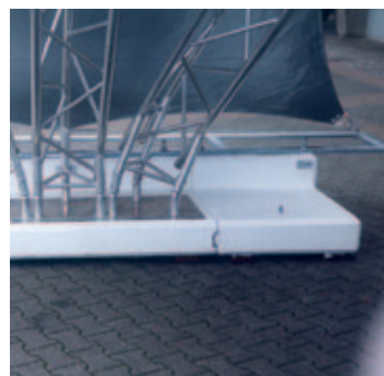
Ballasting by installation on pre-cast concrete
