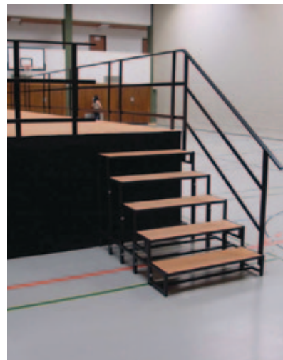
Staircase railings inserted from above
