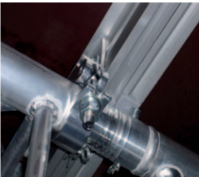
Platform fastening to trusses
