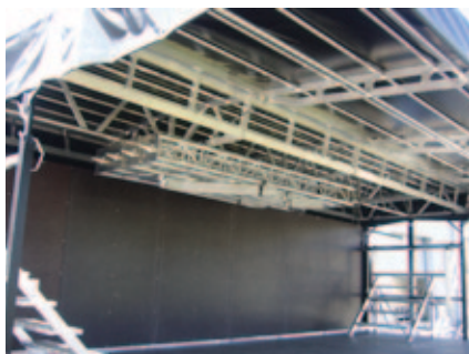
For transport, struts and railings are attached to the roof supports.
