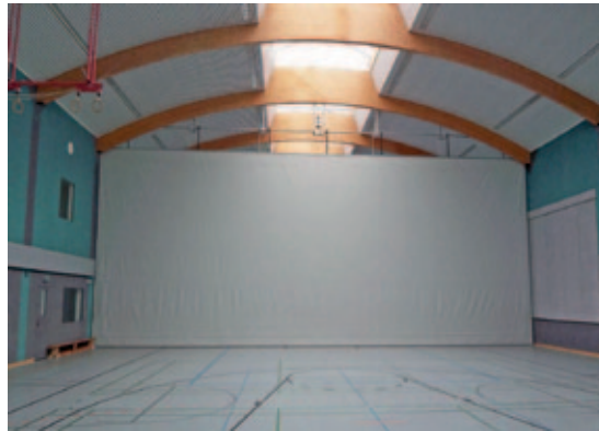
Partitioning curtain mounted on laminated wood truss
