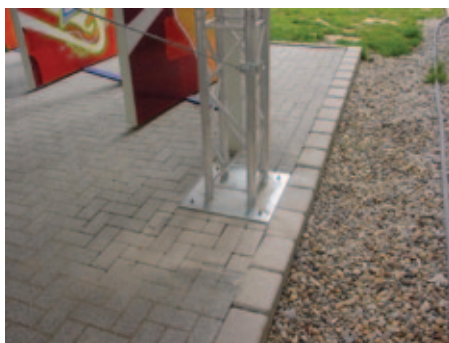
Anchoring to the ground with impact dowels
